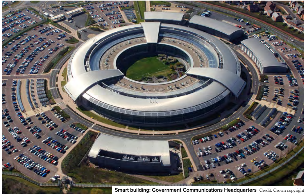
Smart building: Government Communications Headquarters Credit: Crown copyright
