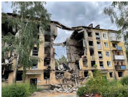
Residencies reduced to ruins: The remains of an apartment block at Antonov Airport, which was struck by a Russian cruise missile on the morning of the 24th February
